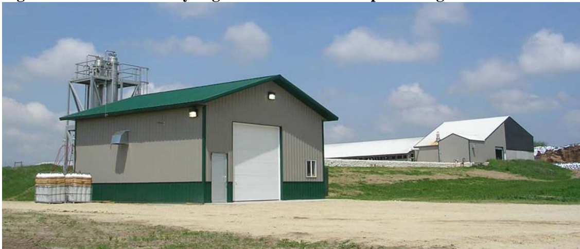
Figure 20 – Emerald Dairy Digester and Gas Cleanup Building
