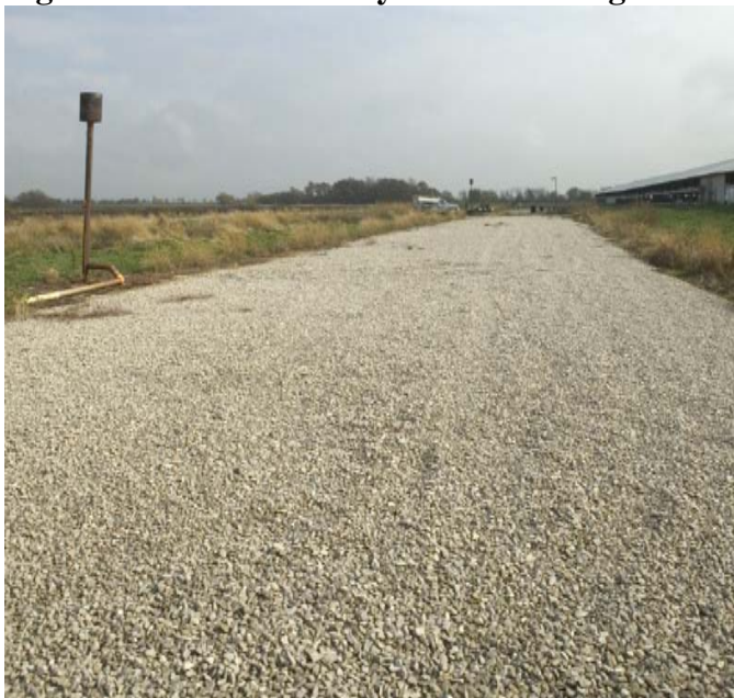
Figure 31 – Holsum Dairy Irish Road Digesters
